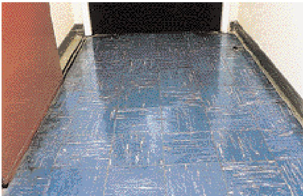
**Asbestos-containing vinyl floor tiles (chrysotile – white asbestos)**
