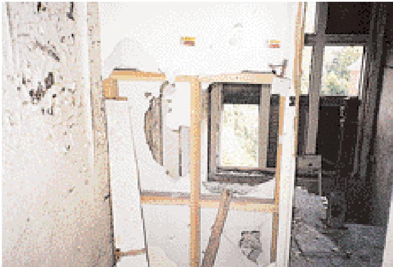
*Damaged asbestos insulating board (AIB) panels containing amosite (brown asbestos)*
