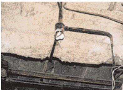
**Sprayed asbestos on steelwork (typically amosite)**
